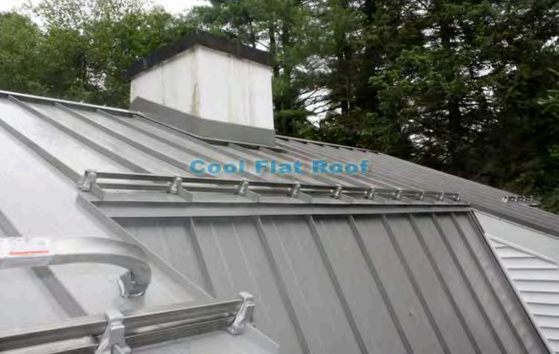
Standing Seam Roof
