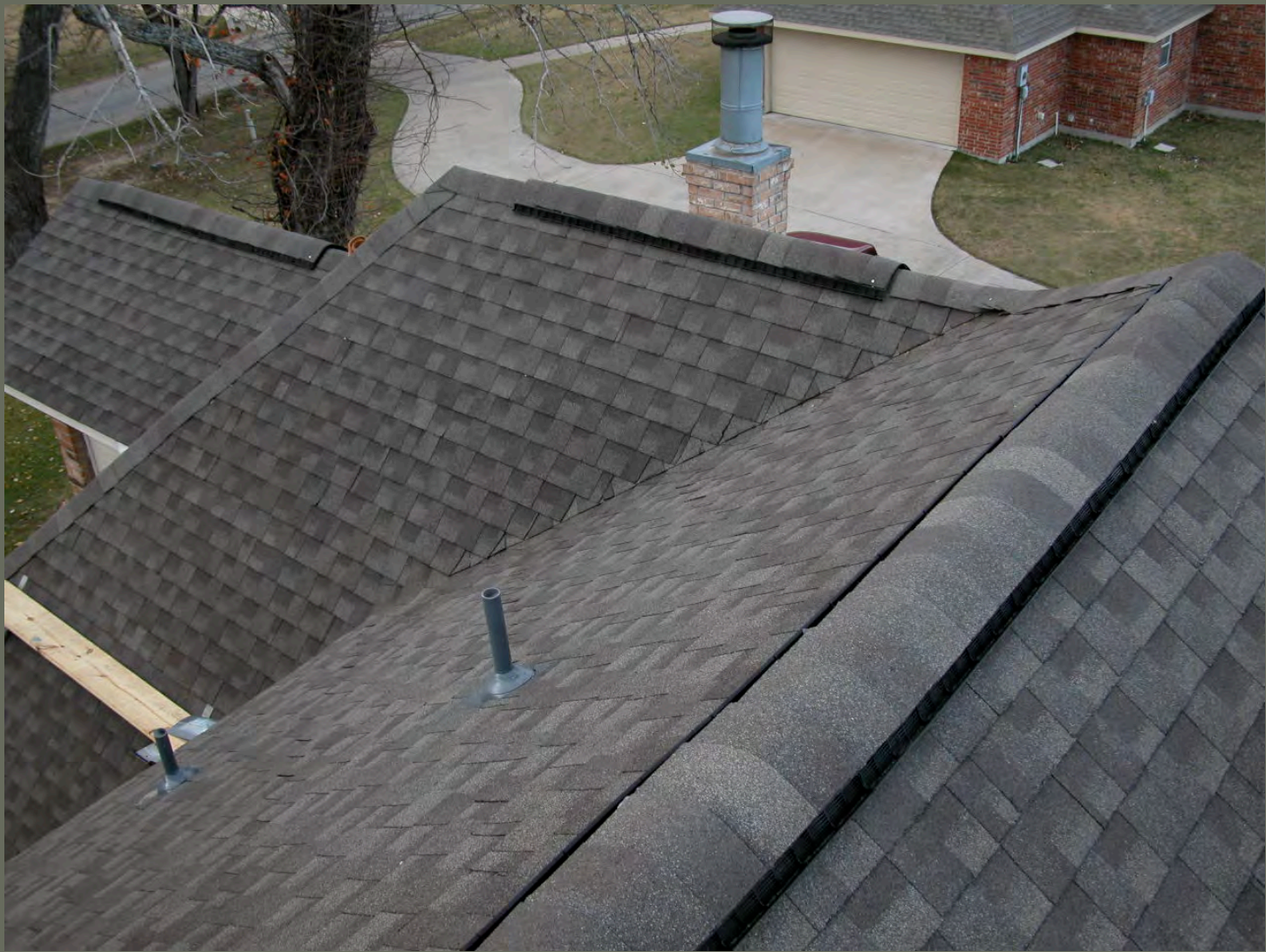
Valley Construction Options: Closed Cut Valley
