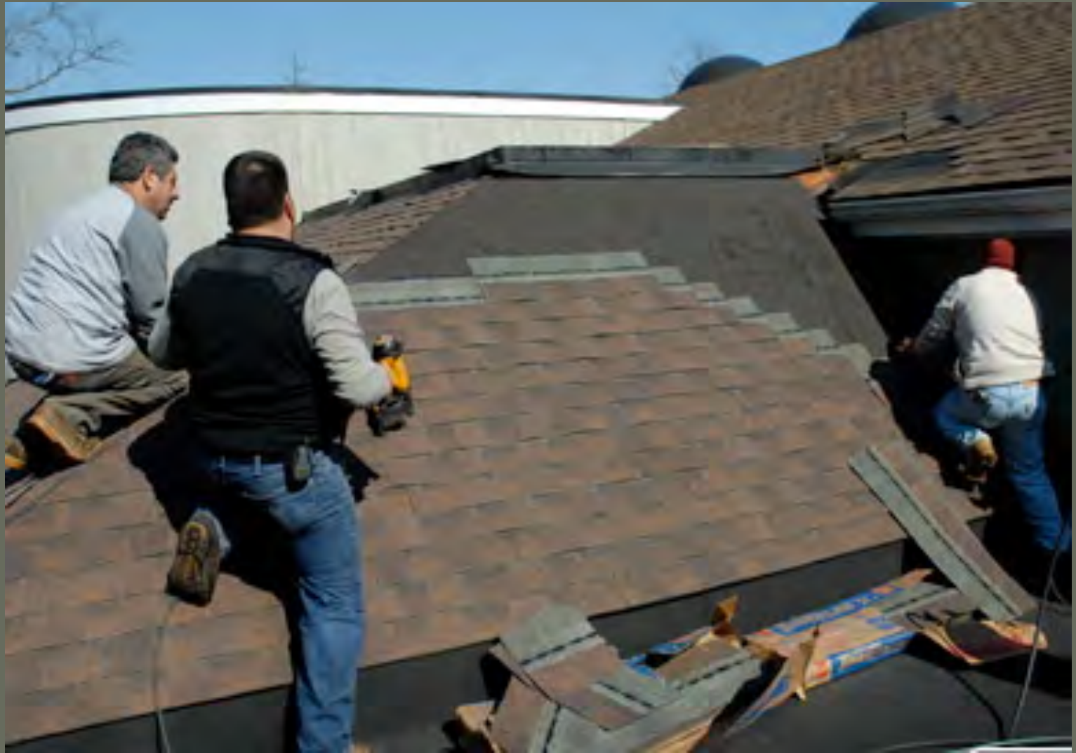
Asphalt Shingle Installation
