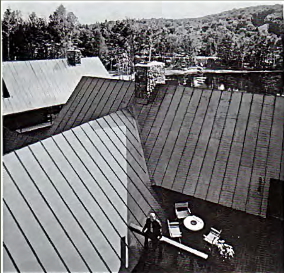
Standing Seam Copper Roof
