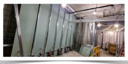
Construction is underway for the Voorhees Bathroom Renovation Project.
