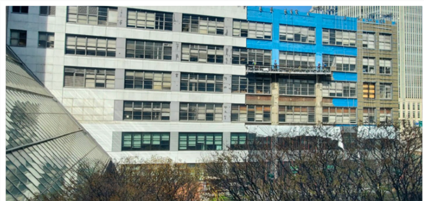
Pearl Building Façade Restoration and Window Replacement project
