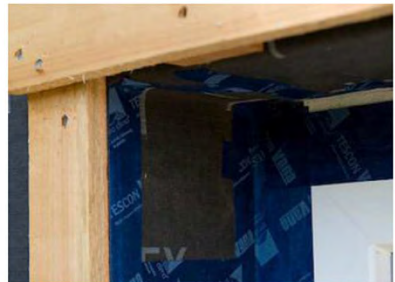
Exterior window with SOLITEX Mento Plus wrapped into rough opening. Taped connections include membrane seams (TESCON Vana) and window frame connections (TESCON Profil).
