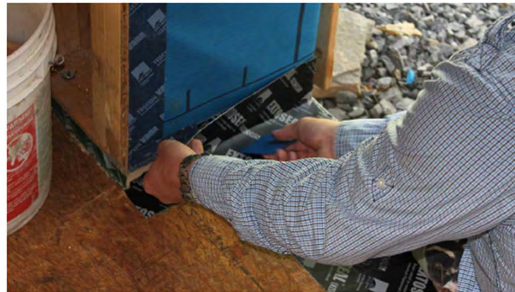
Applying EXTONSEAL Encors and EXTONSEAL Finoc at floor-to-ceiling window (or door). Finoc is used as a capillary break at wall to floor connections. Encors is a self-sealing sill tape for watertight screw/nail penetrations.
