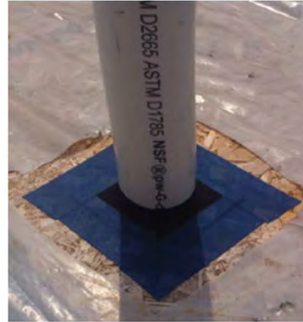
Roflex 50 at roof exterior pipe penetration (left) Roflex 100 at wall exterior pipe penetration containing HVAC lines to be sealed at interior air barrier (right)
