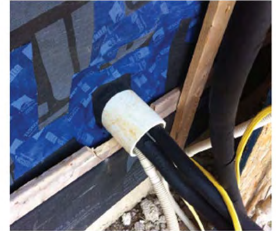
Roflex 50 at roof exterior pipe penetration (left) Roflex 100 at wall exterior pipe penetration containing HVAC lines to be sealed at interior air barrier (right)
