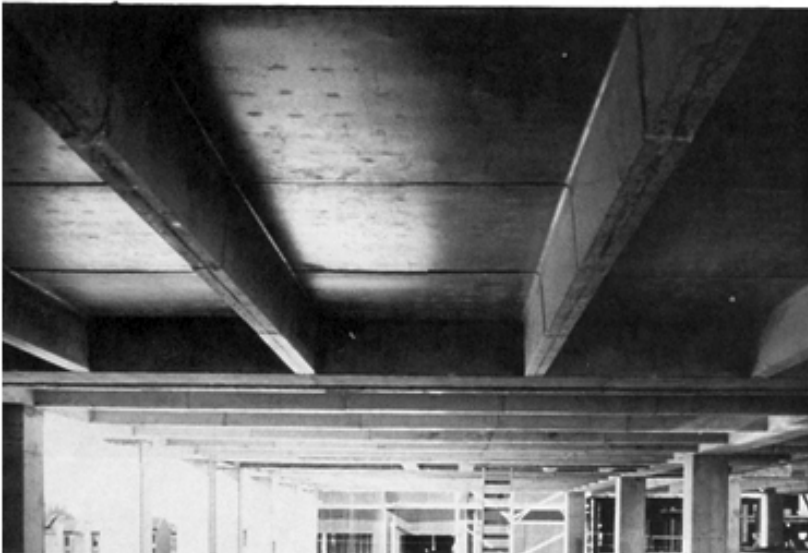
One-way wide module joist system
