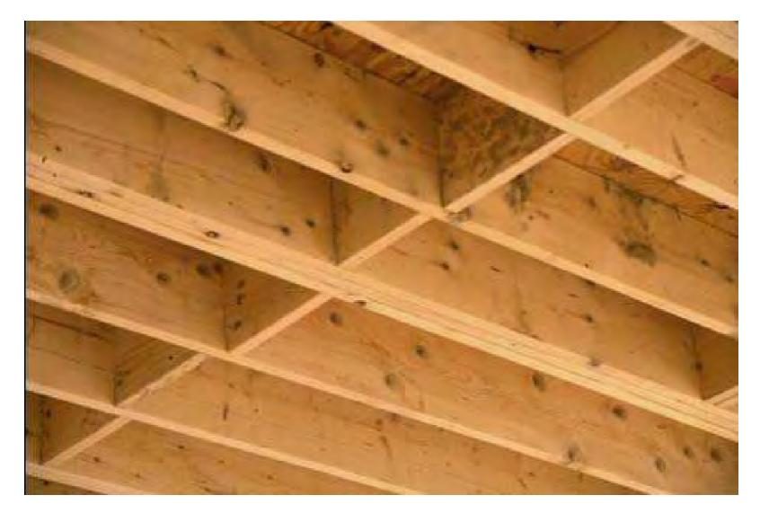
It is necessary to brace long joist at midspan against twisting or buckling. The method being used here is solid blocking with short pieces of floor joist. The blocking is staggered so that the pieces may be end nailed to the joists.
