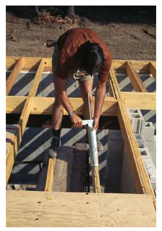
After the floor joist are in place plywood deck is installed on top of them. A mastic adhesive is gunned onto each joist just before the plywood is put down to increase the ridgity of the floor and to prevent squeaks.
