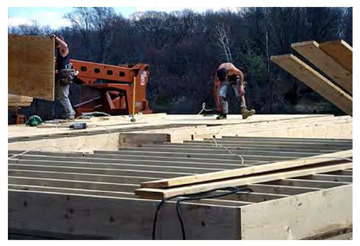
The plywood sheets form the subfloor of the house. The sheets are placed with their long dimension at right angles to the joists and their ends are supported at the mid-line of a joist. An air or electrically powered nailier is used for the nailing.
