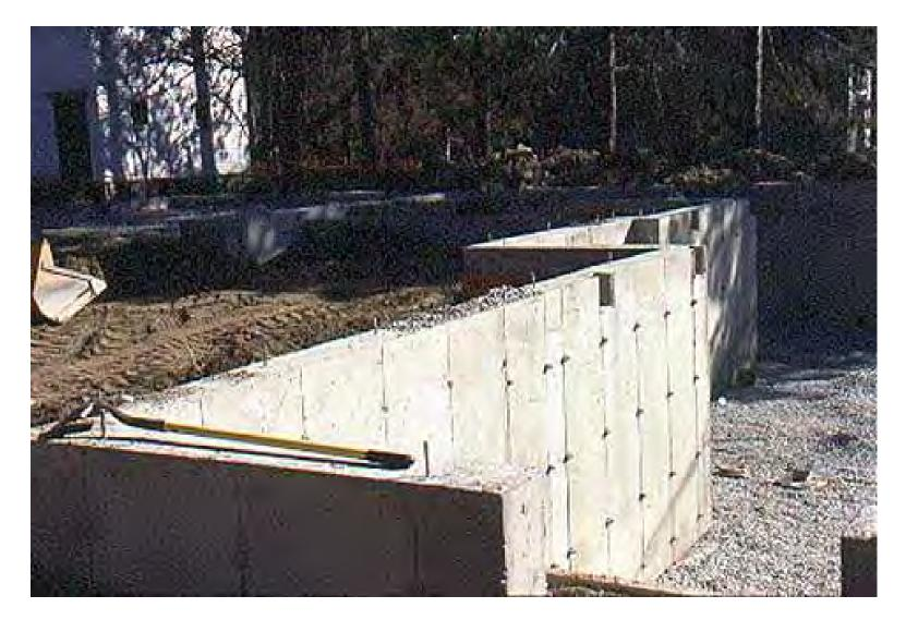
Crushed stone drainage fill has been placed within this foundation wall of a full basement. The vapor barrier and a concrete slab will be added to provide the basement floor. Pockets to receive first floor beams have been blocked out at the top of the wall.
