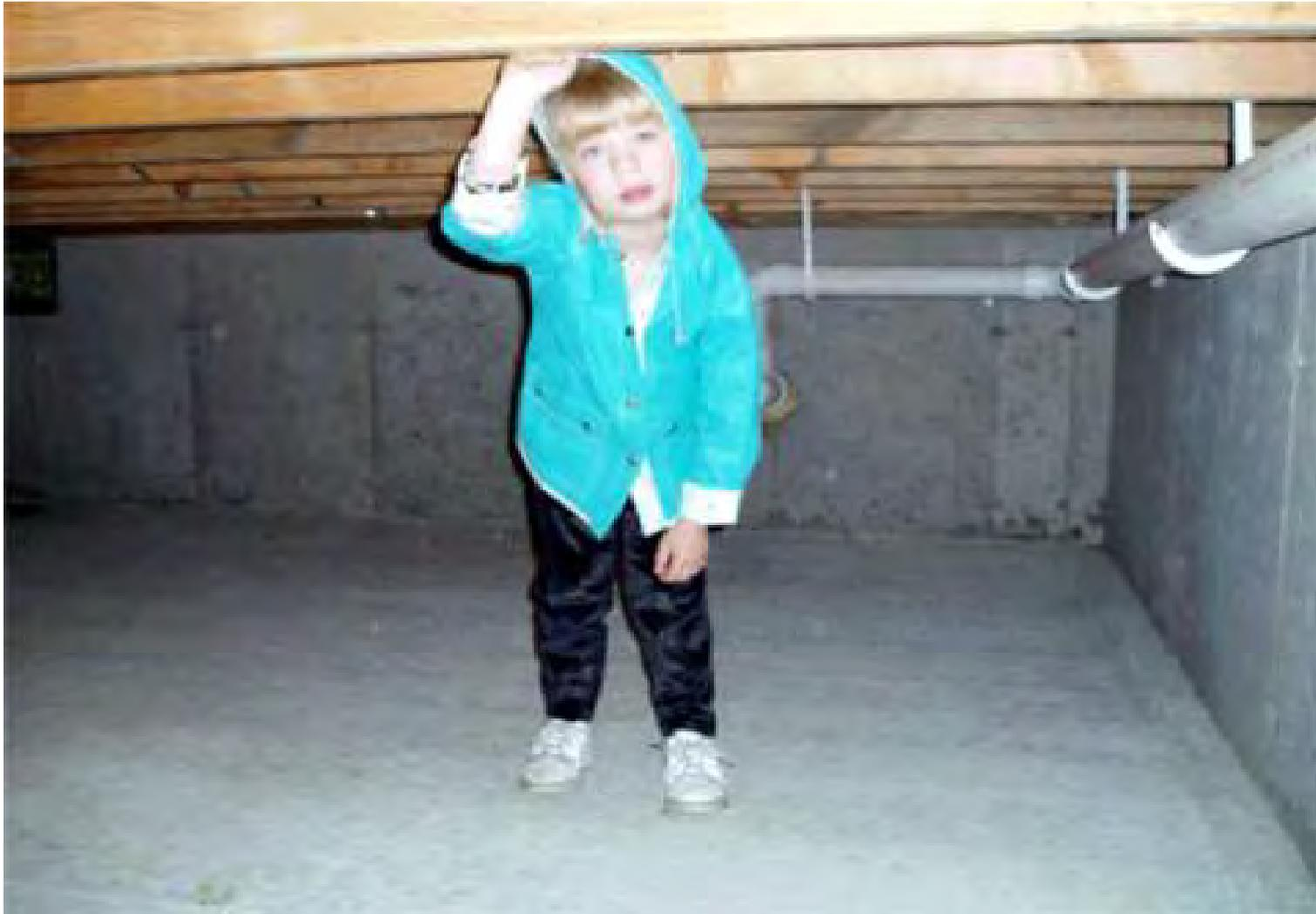
A crawl space isolates the first floor wood platform from the earth and provides space for electrical and plumbing lines. A concrete "rat slab" has been poured over the vapor barrier. The headroom is just sufficient for a small person to stand up.
