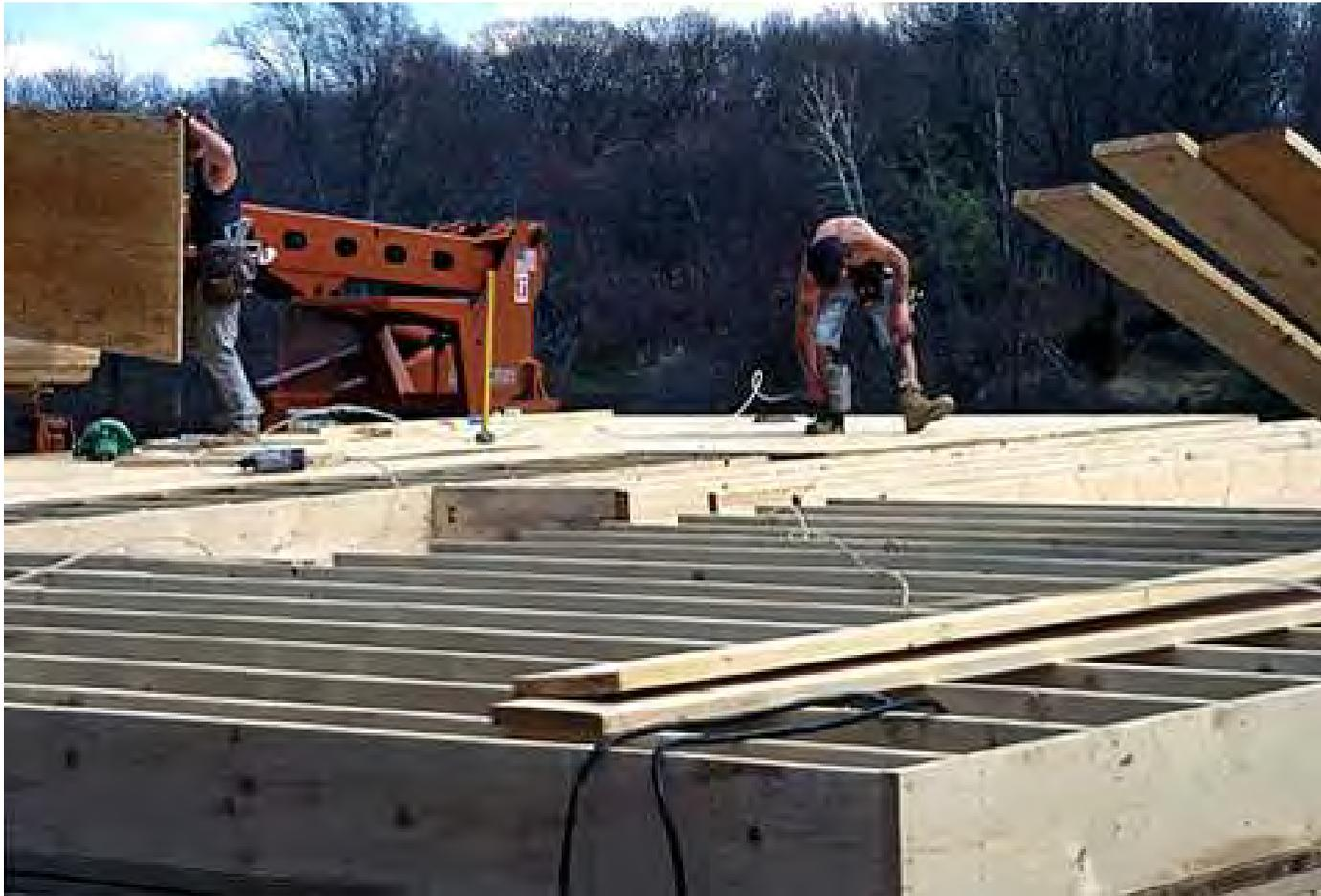
The plywood sheets form the subfloor of the house. The sheets are placed with their long dimension at right angles to the joists and their ends are supported at the mid-line of a joist. An air or electrically powered nailer is used for the nailing.
