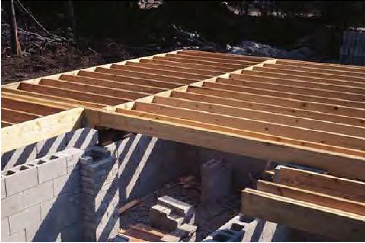
**Some of the interior support for the floor framing is provided by the CMU interior walls of the basement space. Beams made up of triple joists provide other support. Where a partition will fall parallel to the floor joists, and around an opening for a stairway, the joists are doubled.**
