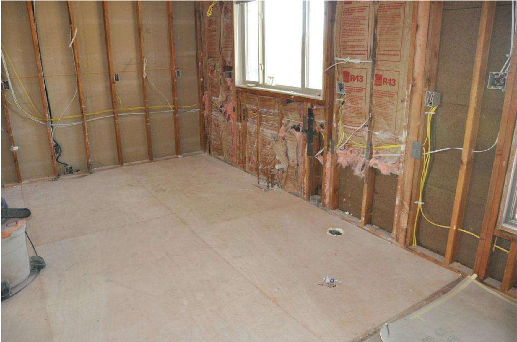
**Plywood:** Plywood subflooring should be installed with its long dimension and face grain perpendicular to the joists. Installing plywood with the subfloor parallel to the joists makes the flooring weaker.
