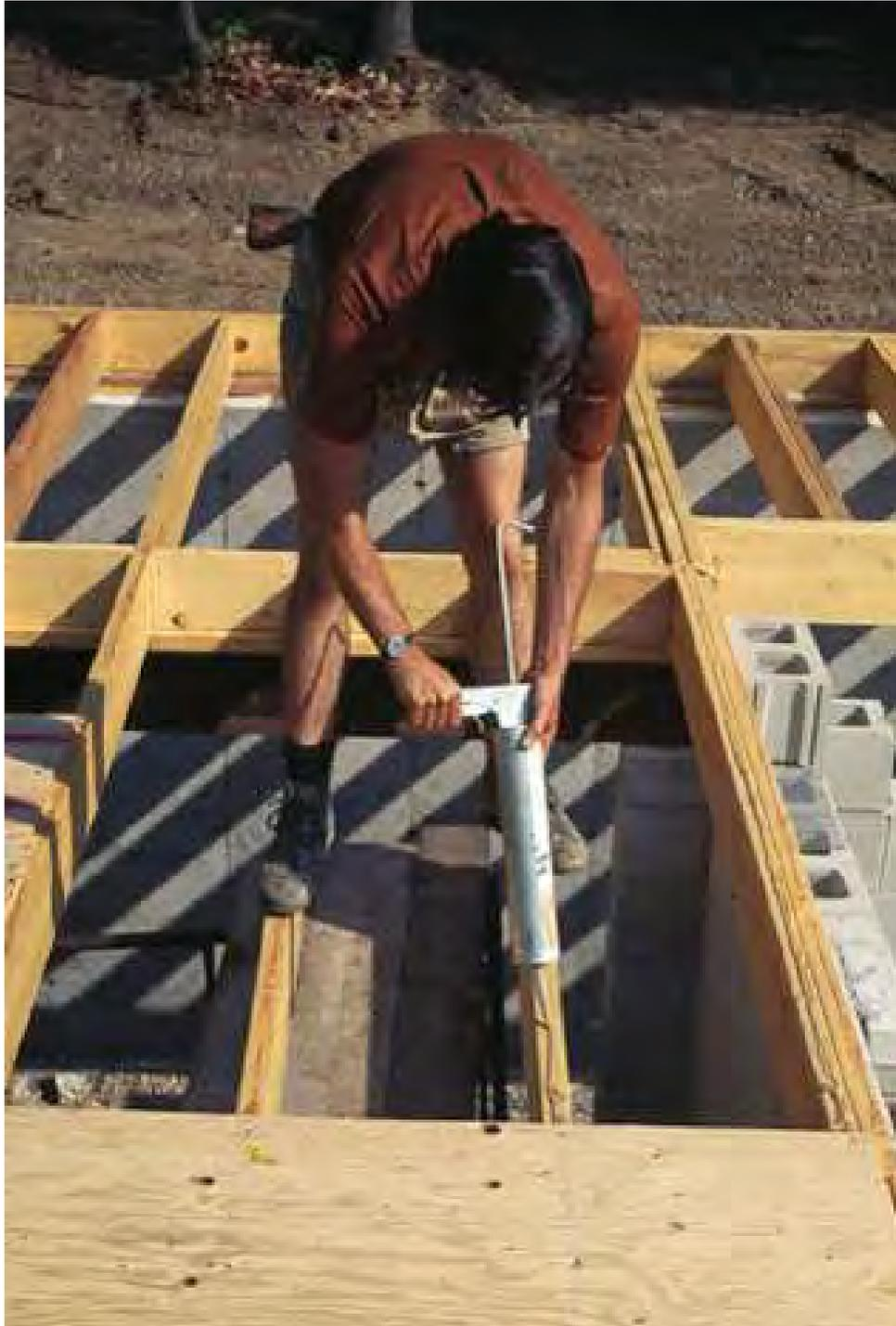
After the floor joist are in place plywood deck is installed on top of them. A mastic adhesive is gunned onto each joist just before the plywood is put down to increase the ridgity of the floor and to prevent squeaks.
