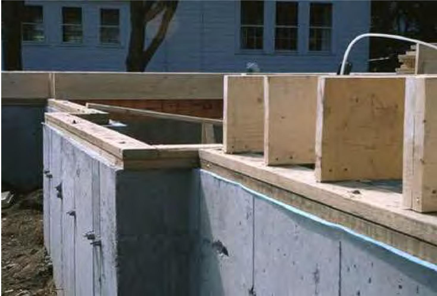
A double 2X6 sill has been secured with anchor bolts and the 2X10 floor joists - 16" o.c. are toe-nailed to them. A strip of sealant is seen between the wood and concrete. Back-filling is not done on the outside of the basement wall until the floor framing is in place to serve as bracing.
