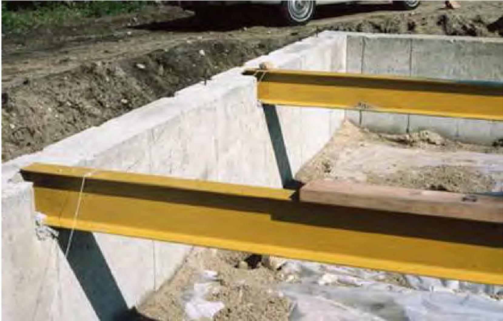
This foundation wall is forming a crawl space. Porous gravel or crushed stone fill is placed on its floor to assure good drainage and a sheet plastic as a vapor barrier is laid on top. Steel beams may support the first floor wood joists.
