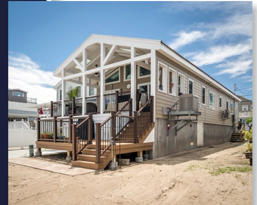
↑ Final view of completed home, resilient, cost effective, and attainable
