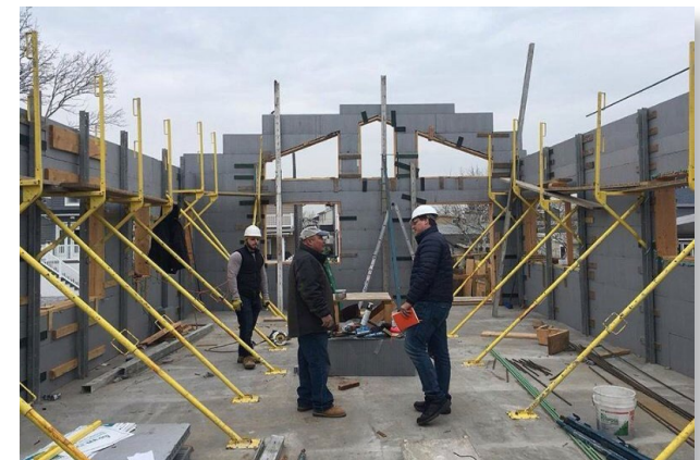
↑ Site meeting reviewing the all-hazard passive house construction process
