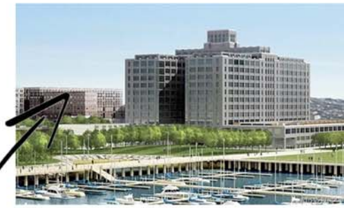
ONE BROOKLYN BRIDGE PARK RESIDENCES
