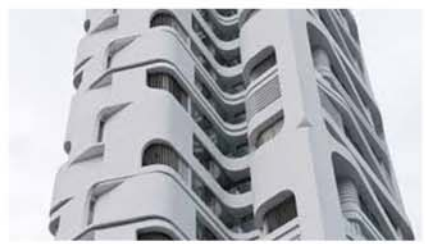
GLASS FIBER REINF.CONCRETE
