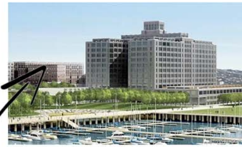
ONE BROOKLYN BRIDGE PARK RESIDENCES
