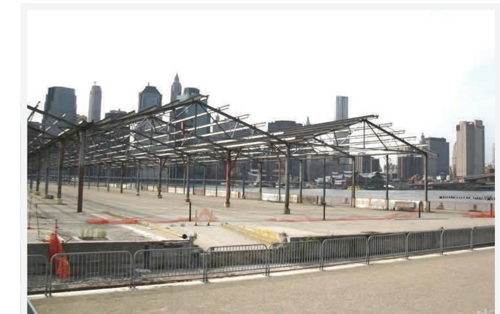
The structural framing of the old warehouse sheds on pier 2 were kept intact to be refitted with a translucent roof acting as a sun and rain shelter.
