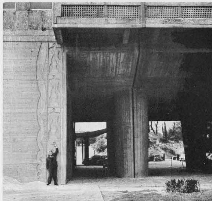
The colossal underpinning of Le Corbusier's Marseille block, four men high See also illustrations page 172
