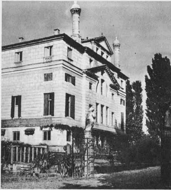
Palladio: Villa Foscari, Malcontenta near Venice. Main entrance façade. The façade design reflects the interior disposition in which a large barrel- vaulted central hall rises to the height of the pediment. The pediment in front corresponds to the loggia on the garden façade shown on the opposite page
