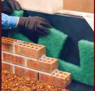
cavity masonry walls
