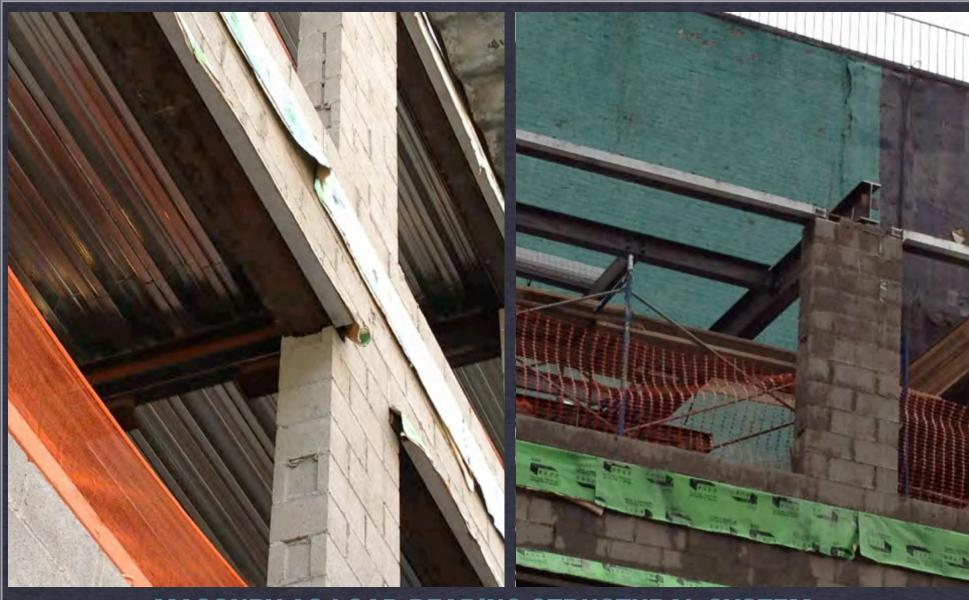
**MASONRY AS LOAD BEARING STRUCTURAL SYSTEM**
