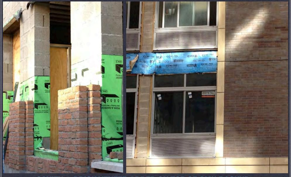
**CAVITY + BRICK VENEER ADDED ON TOP OF CMU BACKUP**
