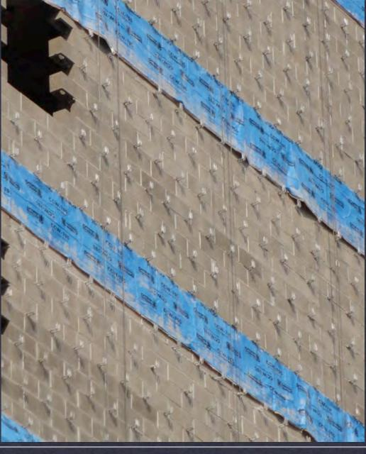
composite cavity masonry walls
