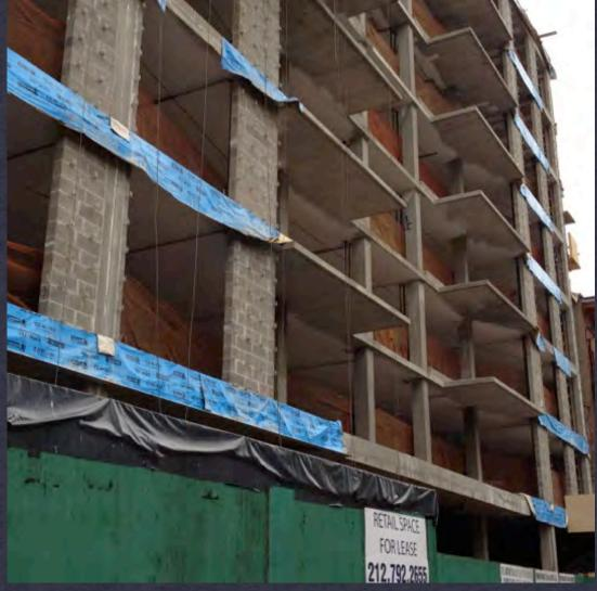
MASONRY AS: INFILL + VENEER WITHIN STRUCTURAL FRAME (NON-STRUCTURAL)
