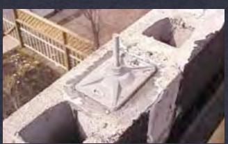
posttensioned masonry walls
