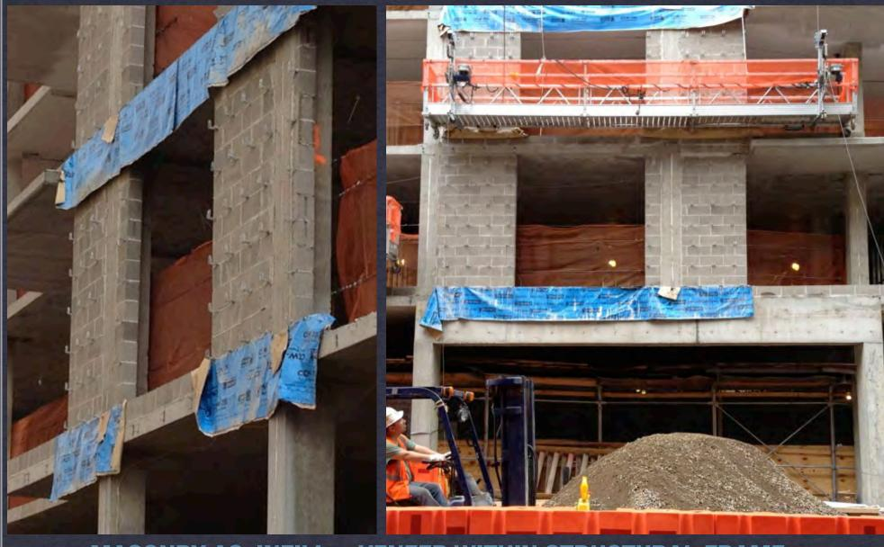
MASONRY AS: INFILL + VENEER WITHIN STRUCTURAL FRAME
