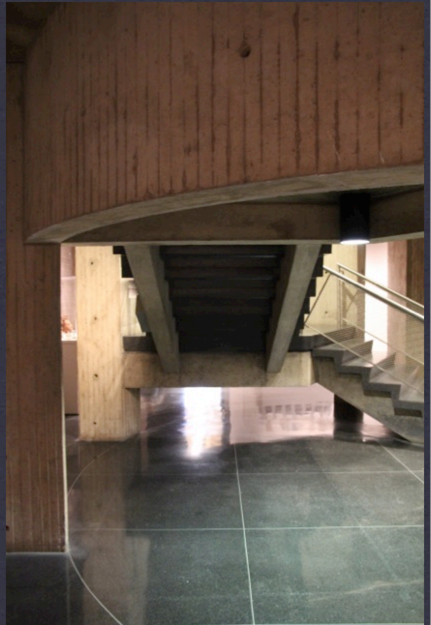
basement level arch 1230
