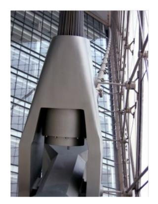
The curtain wall act as greenhouse and warm up the leaving space. The sunlight heat up objects and they give off heat in a form of long-wavelength.
