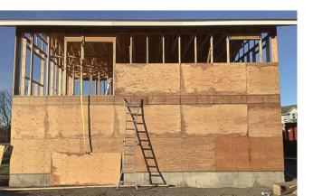
Place exterior sheathing on the exterior of the structure
