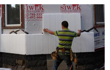
Place exterior insulation on the exterior of the structure
