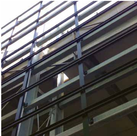
Layout of the Attachment Primary and Secondary attachment L-Bracket
