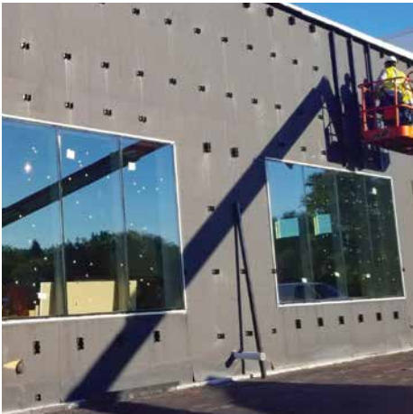
Layout of the Attachment Primary and Secondary attachment L-Bracket
