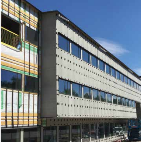
Cut-To-Size Slabs Installed onto the Sub-frame and attached using keil anchors to the Extruded Aluminum Profiles.
