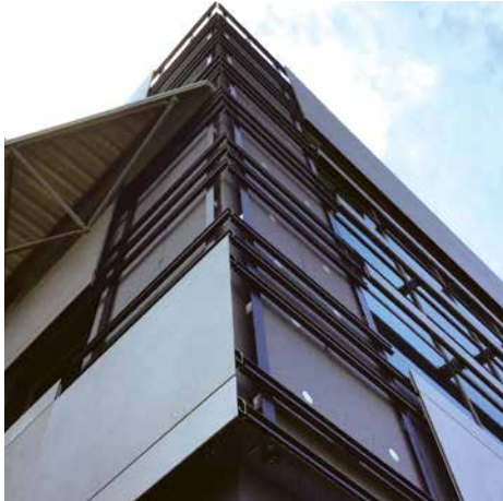
Cut-To-Size Slabs Installed onto the Sub-frame and attached using keil anchors to the Extruded Aluminum Profiles.
