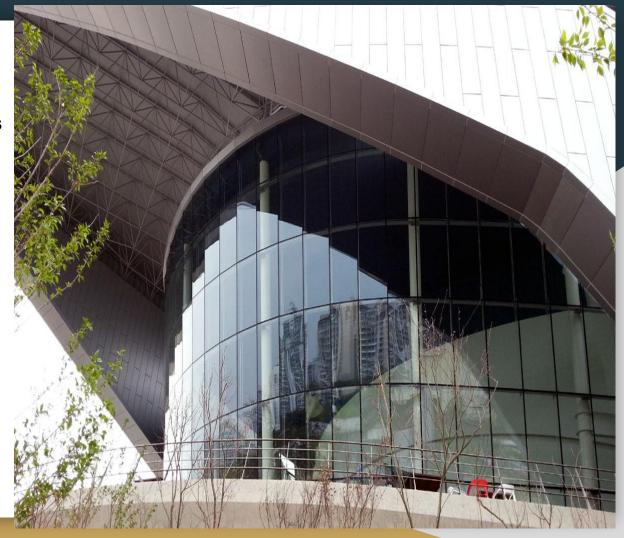
It can be waterproof due to the vacuum space between the two glass sheets is filled with isolators to overcome mechanical pressures and weather conditions.
