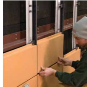
Continue building TerraClad™ courses
