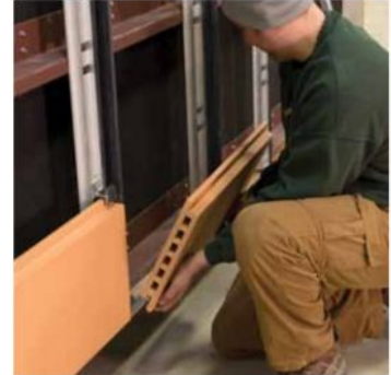
Install TerraClad™ panels
