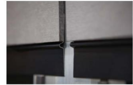
1) Before final fixing of the lowest rivets on a panel, the profile is slid up under the panel.
