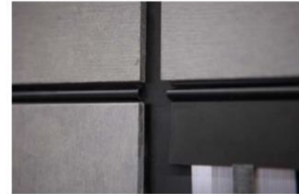
1) Before final fixing of the lowest rivets on a panel, the profile is slid up under the panel.
