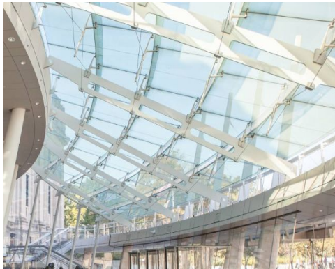
Picture 2: Modernized ceilings
