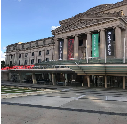
This image captures the "traditional" architectural view
