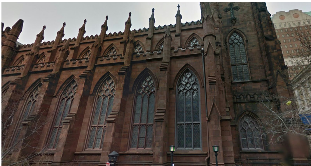
This is the south facing side of the church seen from Clinton St. The brownstone masonry can be seen well in this photograph.
