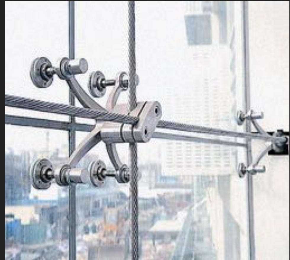
FIX POINT GLASS CURTAIN WALL YEKALON GROUP
