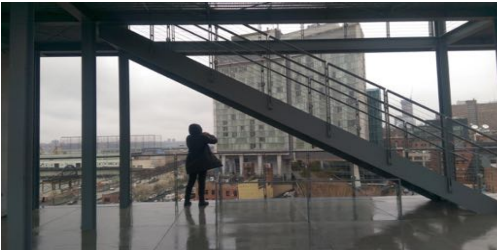
Outdoor stairway (view of Highline)
