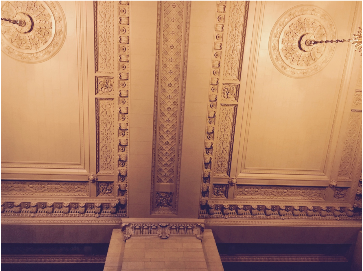
Waiting Room Ceiling at Grand Central Terminal
