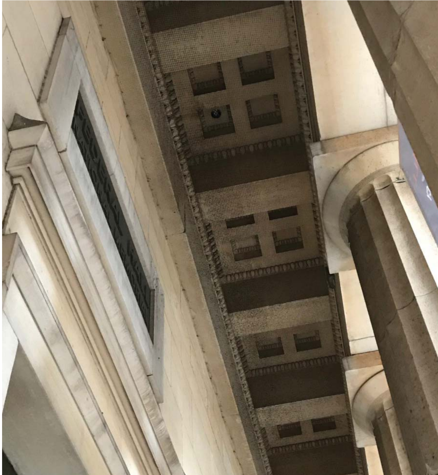
VIEW UP AT ENTRY
