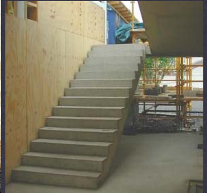
inclined one-way solid slab
