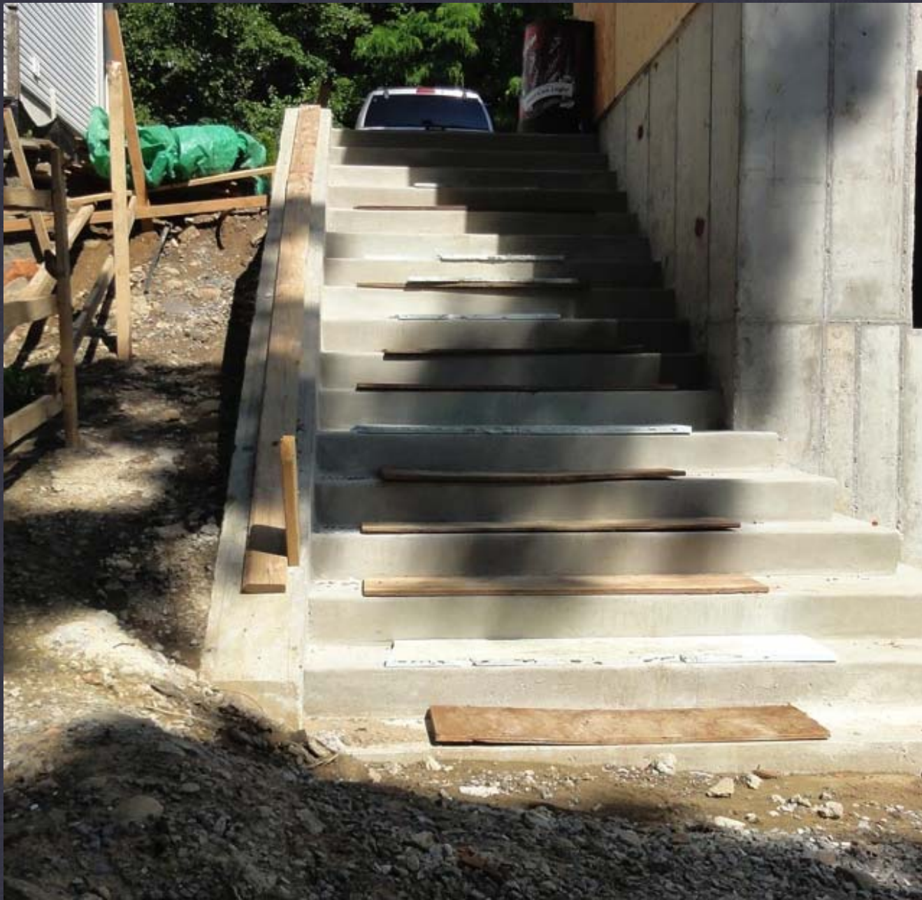
CAST IN PLACE STAIR
